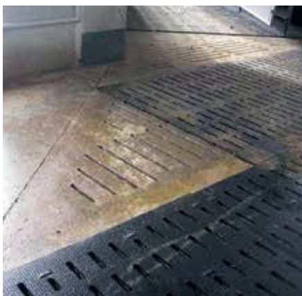
during the installation ...
